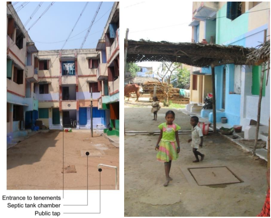
Figure 4: Location of septic tank chambers in PN
