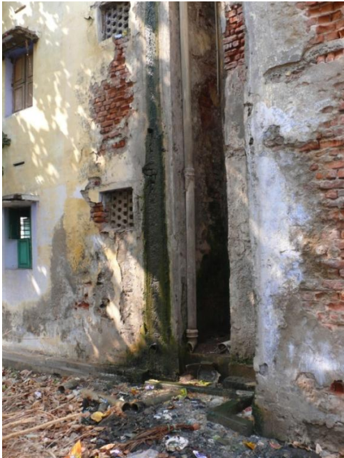
Figure 1: Choked septic tank in the poor performer, SN
