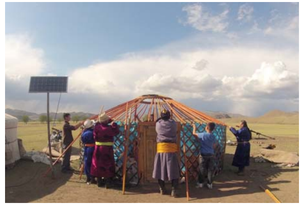
Herders assembling a ger along with solar home system
