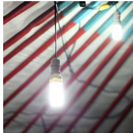
Lights powered by solar electricity Photo credit: Stephan Bachenheimer/World Bank
