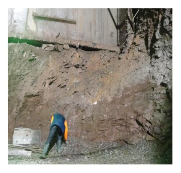
Distressing of the siltstones after excavation, under the concrete struts
