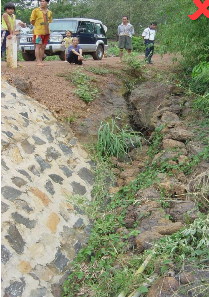
Incomplete drainage work off the Cau Long Binh Bridge
