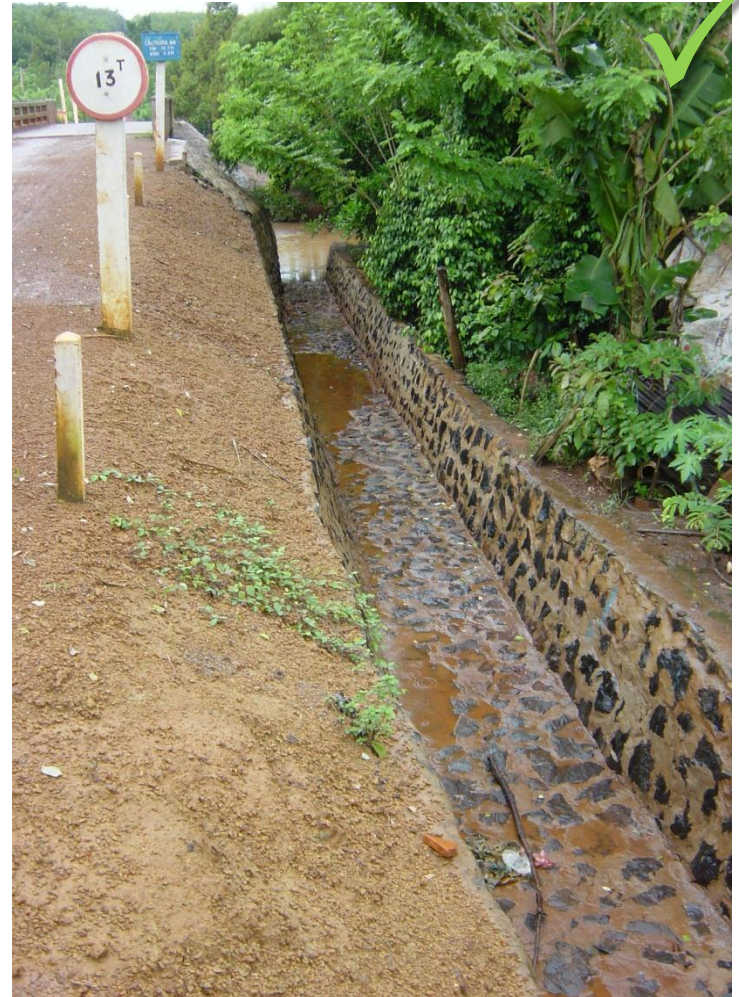
Drainage built according to specifications off the Cau Truong An bridge (Rural Transport Project in Vietnam)
