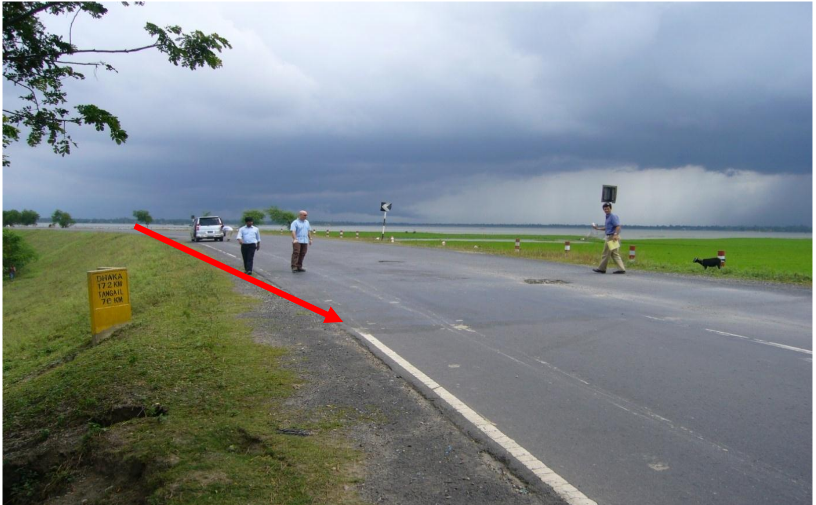
Different companies built components of this major toll road project (Road Rehabilitation and Maintenance Project in SAR)
