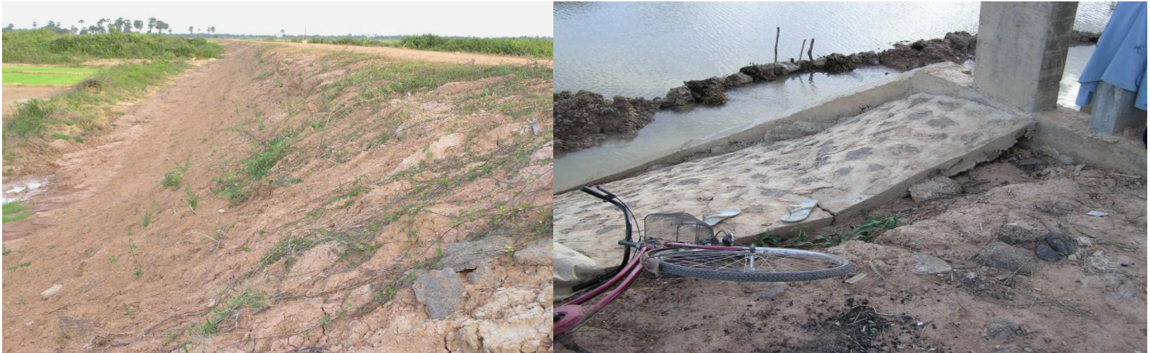
The earth bund shows erosion after only three months...
