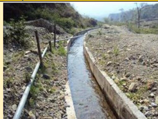
Irrigation canal at Bigante irrigation, Pokhara
