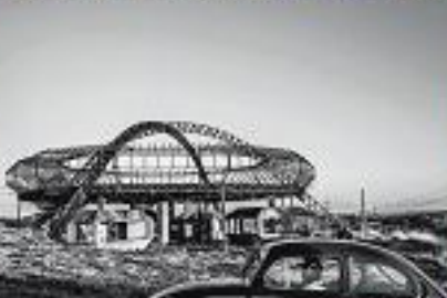
View of a new building in a state of ruin in Brazil.
