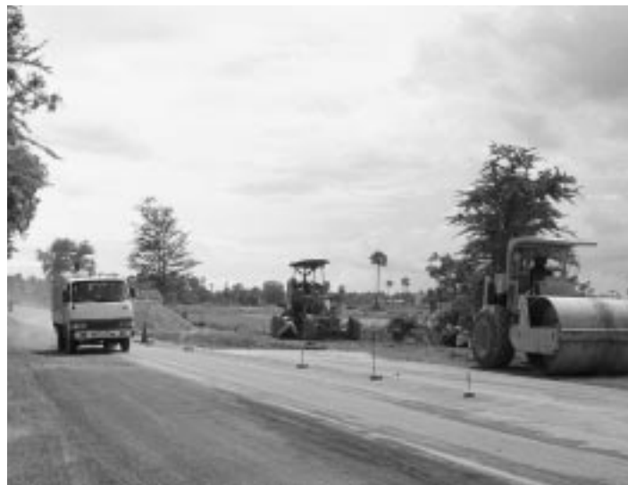
Road construction in Cambodia.
