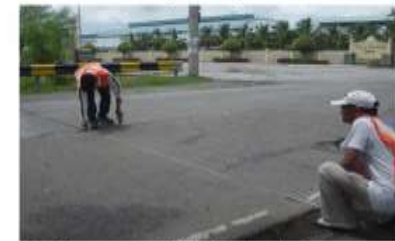
2. Measure width of affected area
