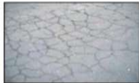
Fatigue (Alligator) Cracks
