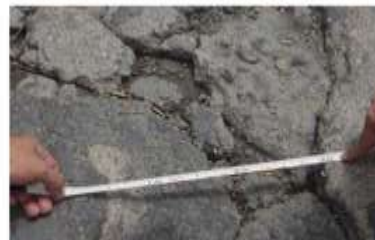
4. Measure largest width of crack
