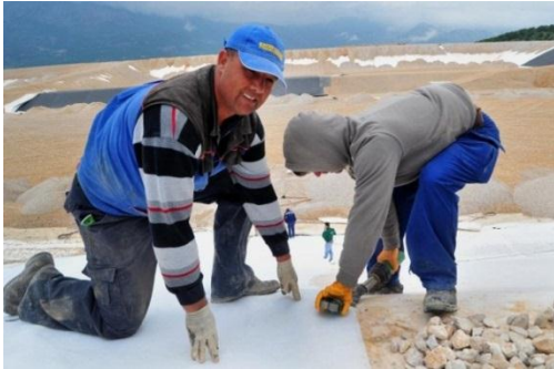
Picture 1. Sanitary Landfill “Možura” Completed in 2012 and expected to operate for 25–30 years
