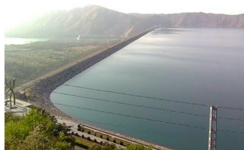
An Overview of Tarbela Dam
