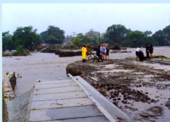
Figure 3.6 Isolation of downtown Estelí due to severe damages to a bridge.
