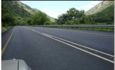
N4 ROAD ON THE MAPUTO CORRIDOR AFTER CONCESSION
